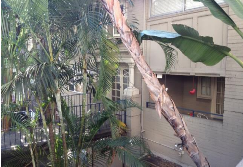
View of: No. 173 Walker street Looking North east Inspected on: 03.12.2018
