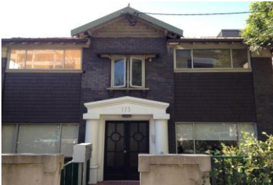
View of: No. 175 Walker Street Looking: East Inspected on: 03.12.2018
