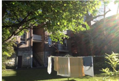
View of: No. 179 Walker Street, rear backyard Looking North west Inspected on: 03.12.2018
