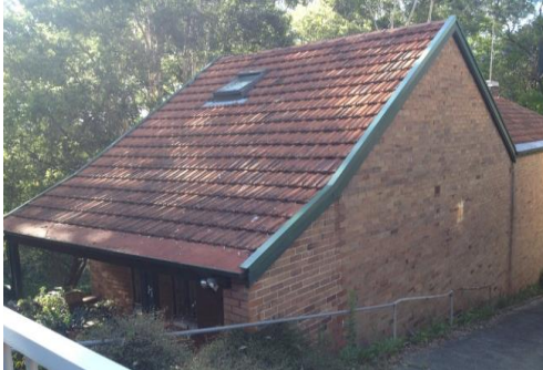
View of: No. 17 Hampden street Looking: North east Inspected on: 03.12.2018
