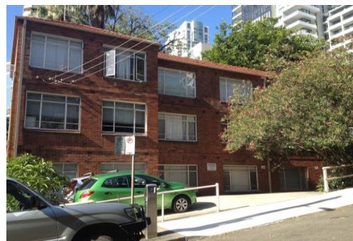
View of: No.11 Hampden Street Looking : North Inspected on: 03.12.2018
