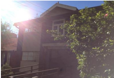
View of: No. 177 Walker Street Looking: East Inspected on: 03.12.2018
