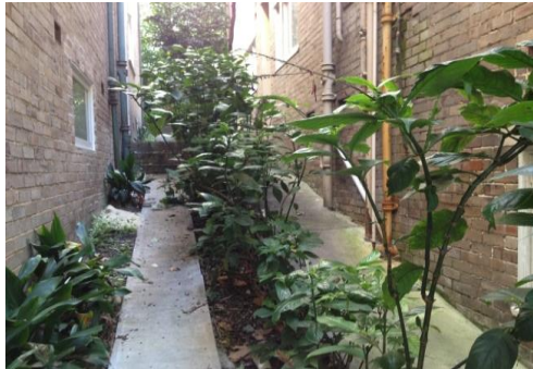
View of: Concrete footpath Looking West Inspected on: 03.12.2018
