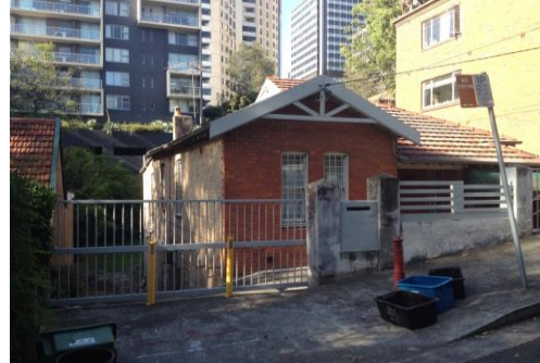
View of: No. 15 Hampden Street Looking North west Inspected on: 03.12.2018
