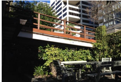
View of: Pedestrian bridge Looking West Inspected on: 03.12.2018
